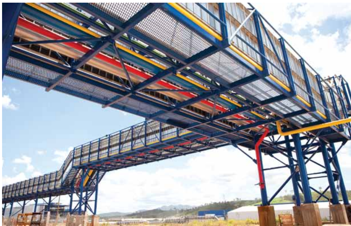
› Pipe Rack – Vallourec & Sumitomo Tubos do Brasil
